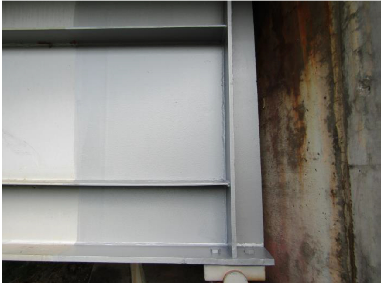
Figure 6: Photograph showing the beam end after it has been recoated
